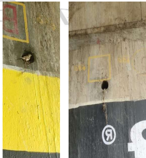
Beam of an underpass with nest of house swift
